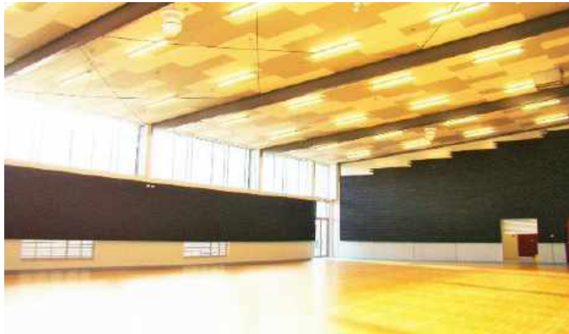
Figure 6: Example of assembly hall / gym – note absorption on ceiling and walls
