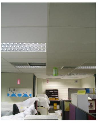
Above: 1/2 completed ceiling, new Sonatex finish applied top left with 12 year old rockwool ceiling panels top right
