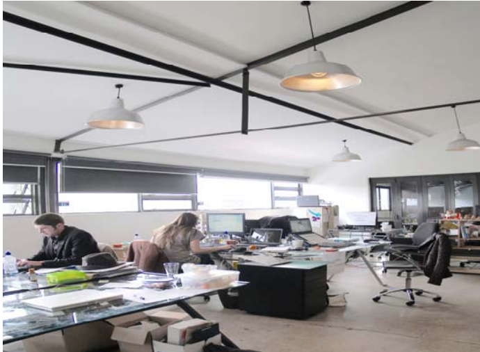
Running with Scissors, Auckland. Triton 50, 2400 x 1200 panels direct fixed over plasterboard lining.
